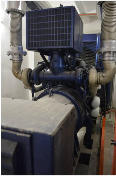
Figure 4.17 Diesel Generator
