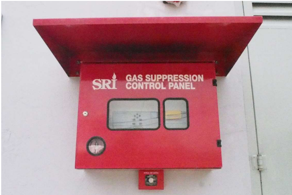
Figure 2.35: Gas Suppression Control Panel
