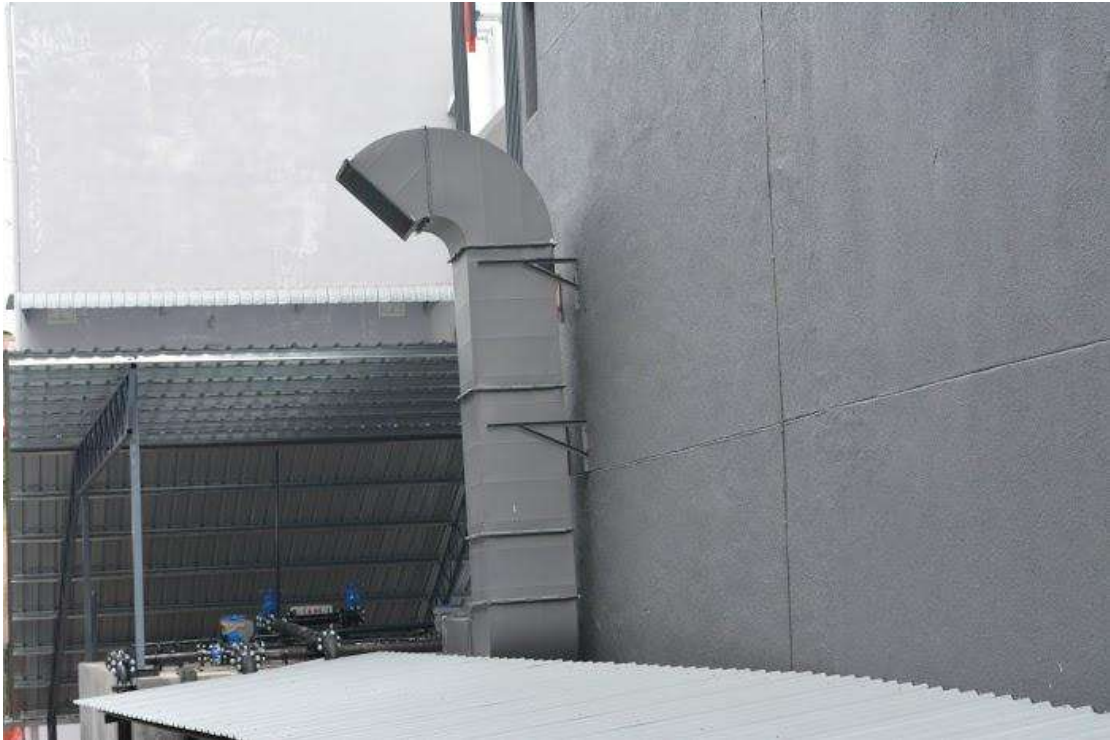
Figure 3.2 Ductwork on Building Exterior
