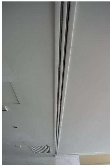
Figure 3.4 Linear Diffuser
