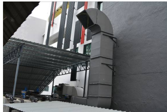
Figure 4.15 Exhaust from kitchen
