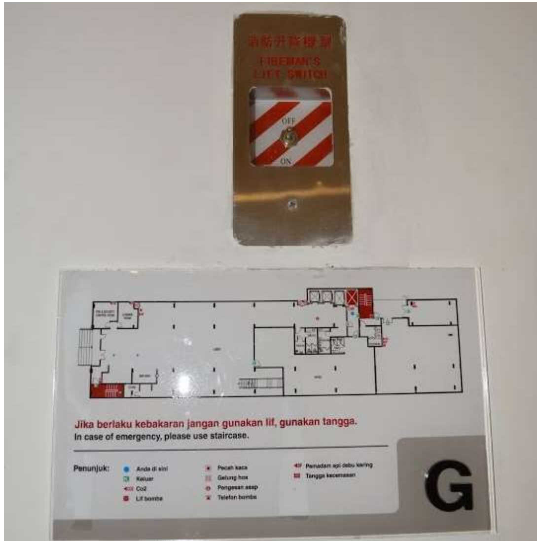
Figure 5.8 Fireman's Lift Switch on the ground floor
