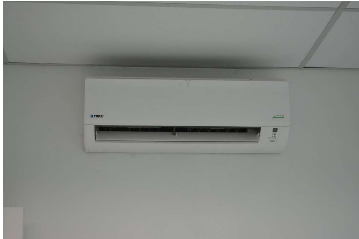
Figure 3.7 Wall Mounted Indoor Unit
