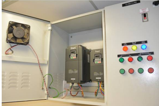
Figure 4.14 Control Panel for balanced system in kitchen
