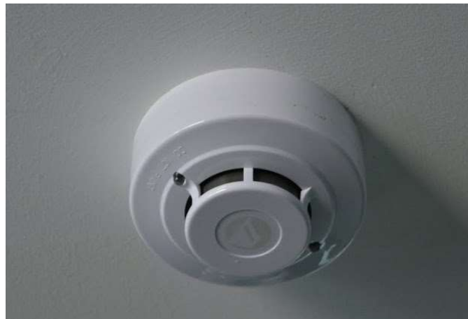
Figure 2.2: Smoke Detector
