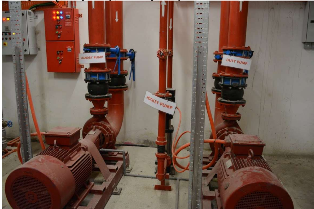
Figure 2.26: Standby Pump, Jockey Pump, Duty Pump
