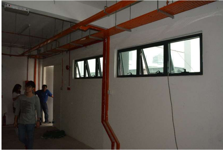
Figure 4.28 Natural Ventilation in Lift Motor Room
