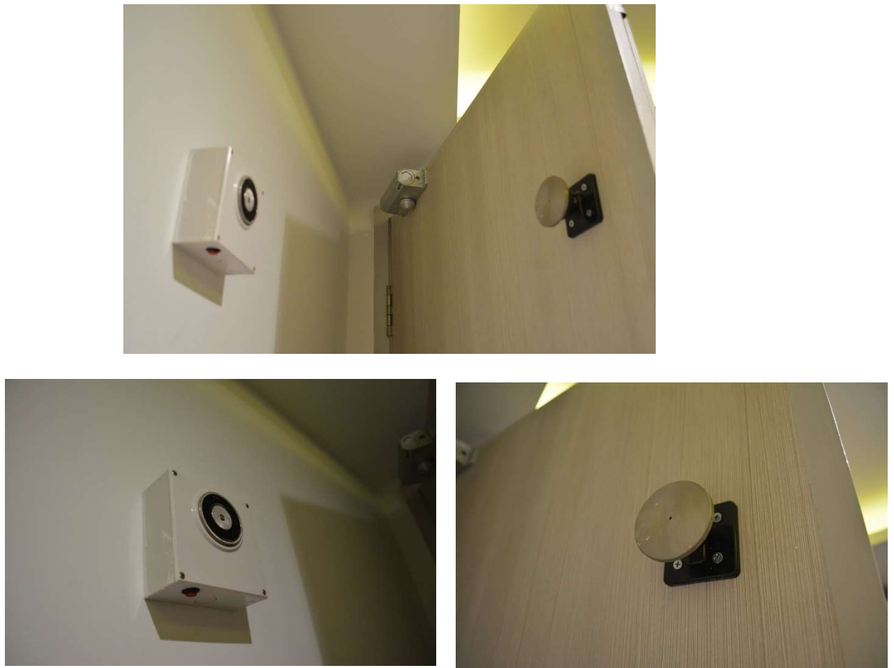
Figure 2.53: Fire Door Closing System
