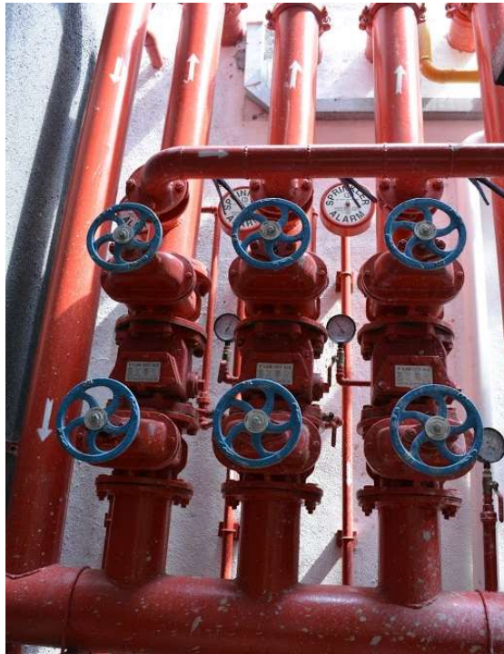
Figure 2.28: Alarm Gong System
