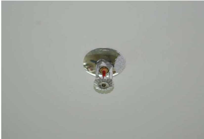
Figure 2.31: Recessed Pendant Sprinkler
