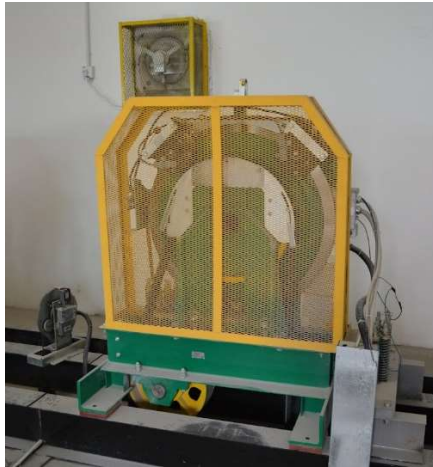
Figure 5.20 Geared traction machine
