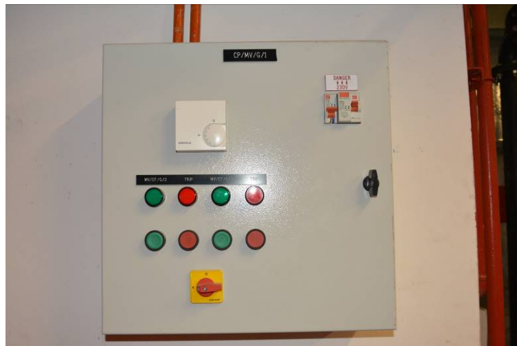
Figure 4.22 Control Panel with temperature sensor
