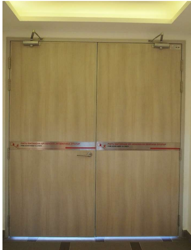
Figure 2.43: Fire Rated Door
