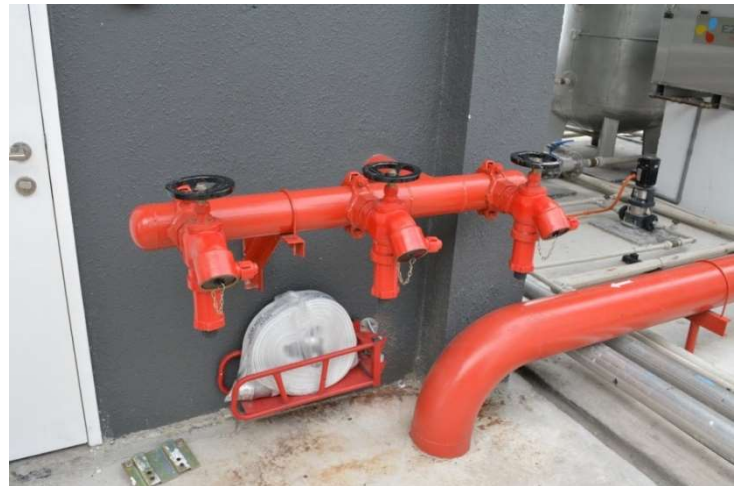
Figure 2.29: Wet Riser and Hose Reel System
