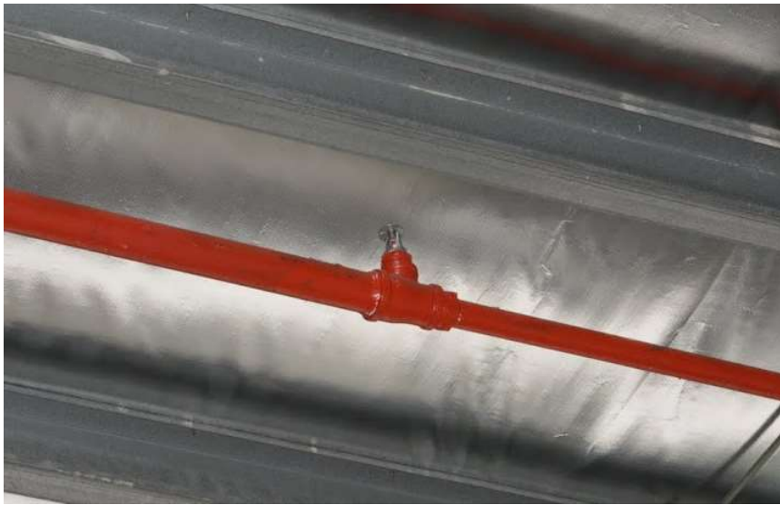
Figure 2.30: Upright Sprinkler
