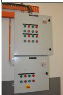
Figure 4.13 Pressurized System Control Panel
