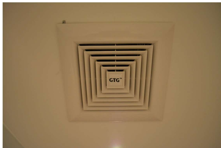
Figure 3.8 Ceiling Mounted Indoor Unit in the Individual Hotel Rooms
