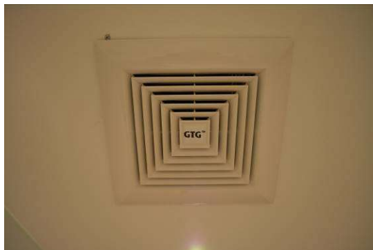
Figure 4.24 Diffuser in toilet
