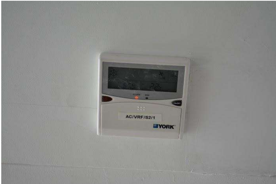
Figure 3.3 Indoor Unit Controller
