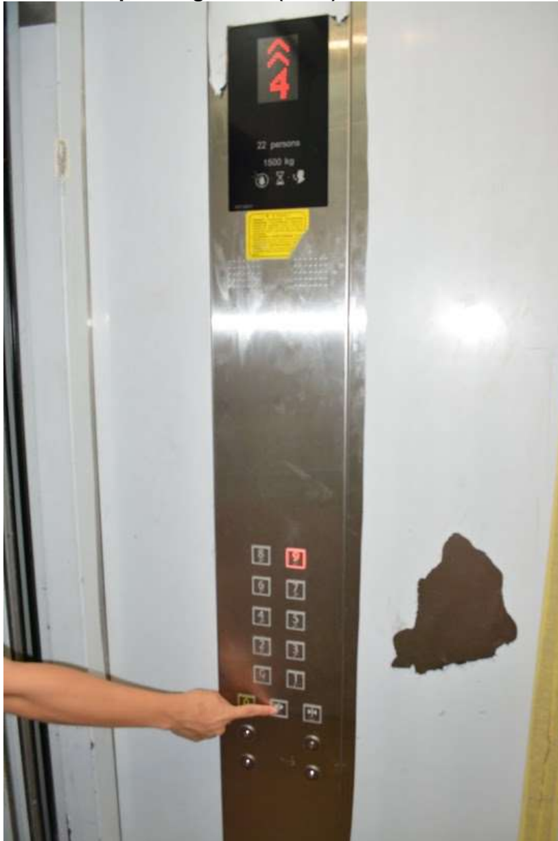
Figure 5.10 COP in fireman's lift
