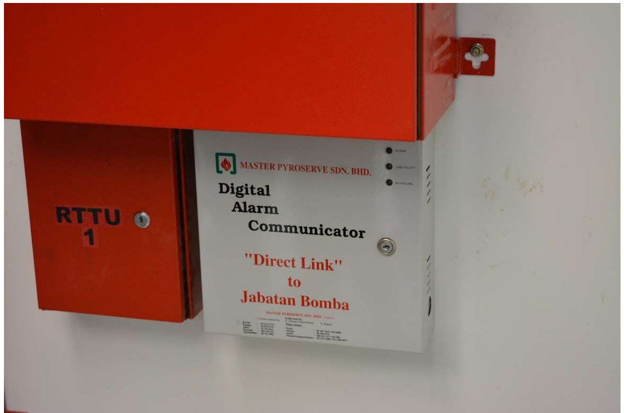
Figure 2.18: Digital Alarm Communicator
