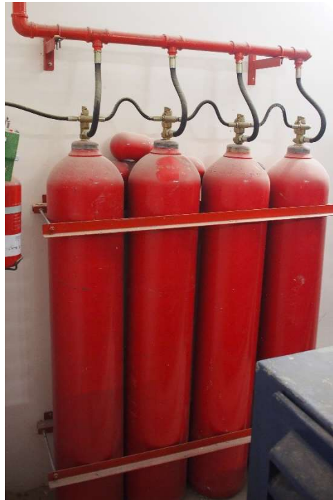
Figure 2.33: Carbon Dioxide Suppression System
