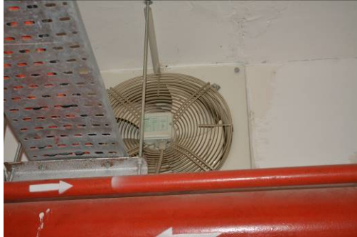
Figure 4.20 Propeller fan
