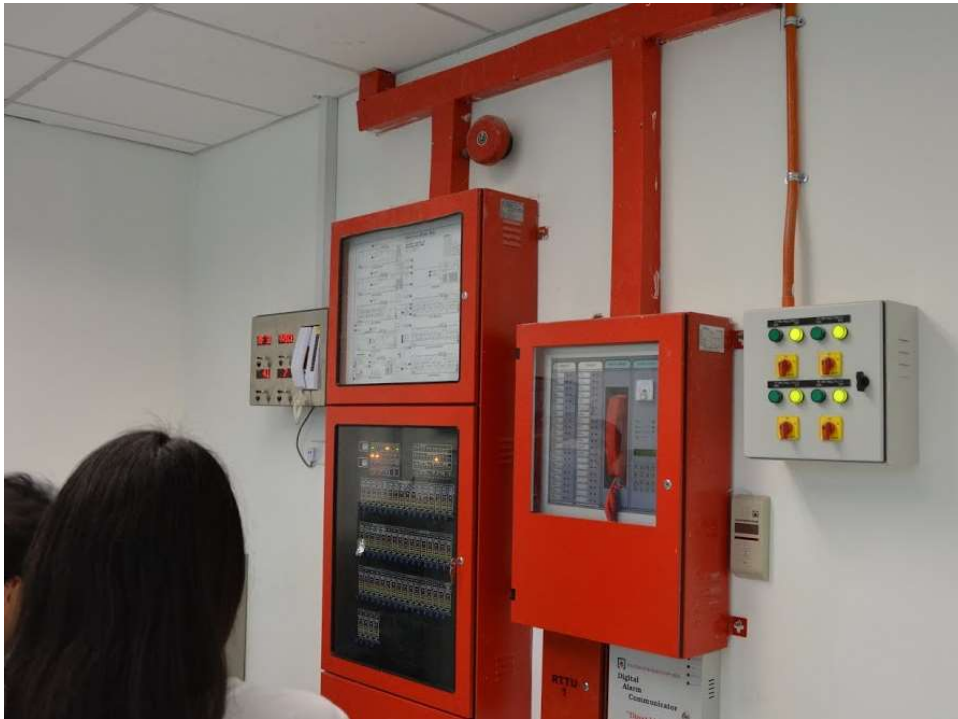
Figure 2.16: Fire Alarm Panel
