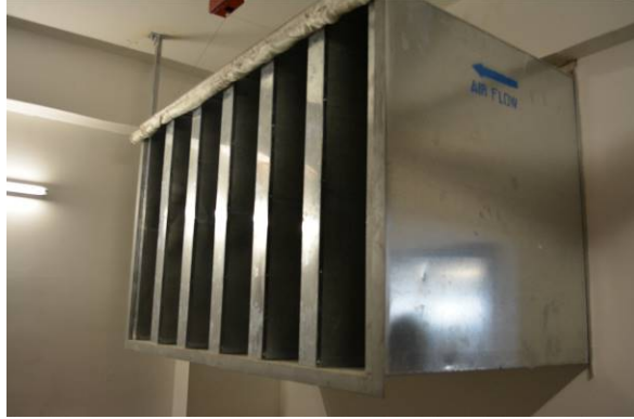
Figure 4.18 Air intake diffuser
