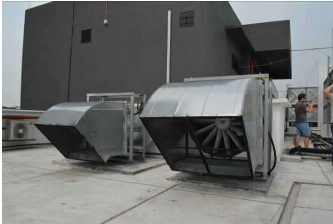
Figure 4.10 Fan to pump in air
