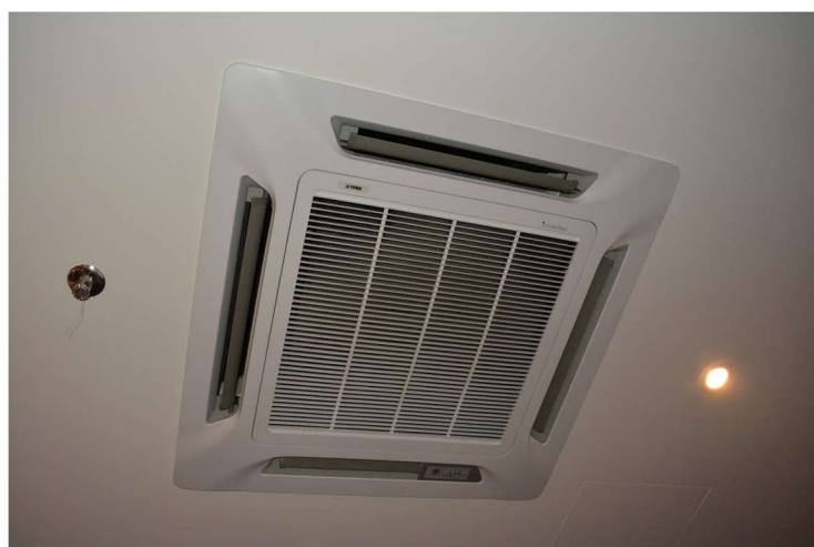
Figure 3.9 Ceiling Mounted Indoor Unit
