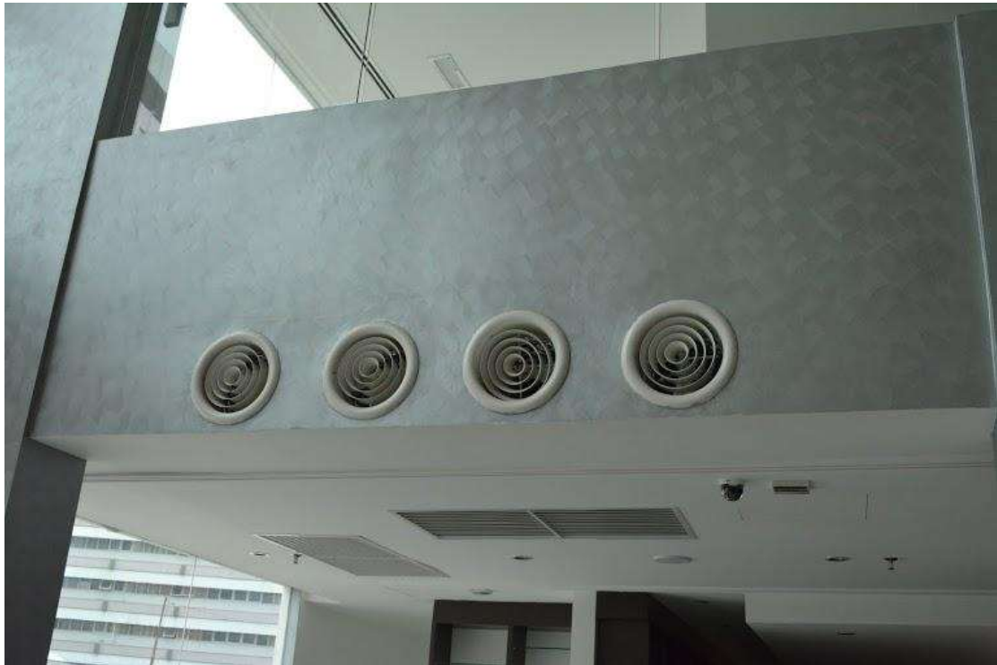
Figure 3.5 Round Diffuser
