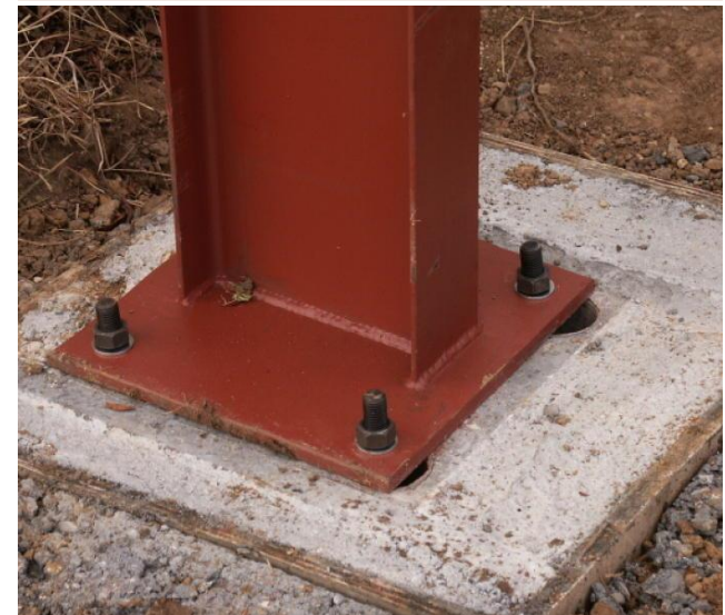
Foundation connection detail
